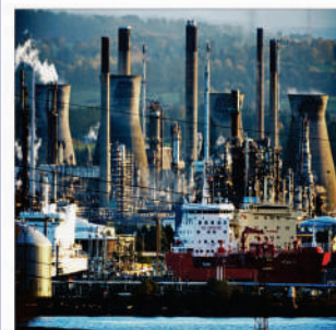
Refinery Petrochemical Plant
